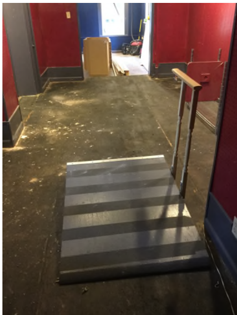
Red Room looking to front room
