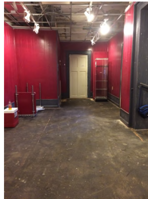
Red Room ceiling tiles and carpet removed
