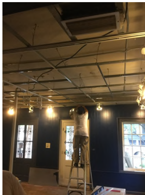
Ceiling tile grid being installed, walls primed.
