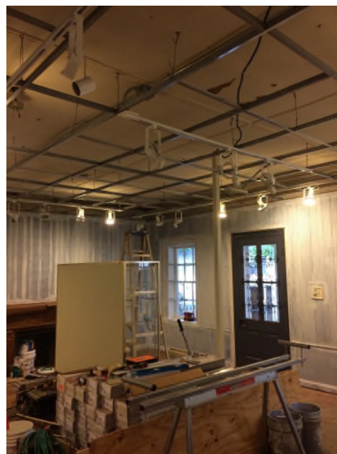
Ceiling tile grid being installed, walls primed.
