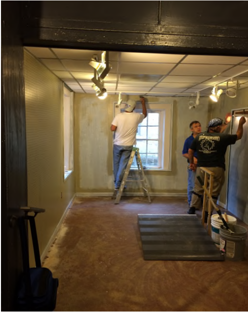
Painting in progress
