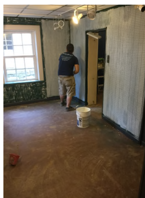
Walls being primed
